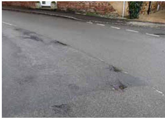
A veritable pothole factory in Church Street in January 2019. Cyclists beware! It doesn't look like they've been marked for filling, but they're forming along seams between different surfaces. Spratton Road, Northampton Road and Creaton Road are all in need of repair - along with the rest!
